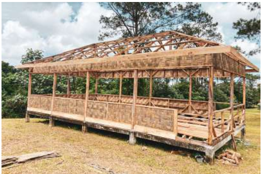
Multifunctional auditorium before completion
