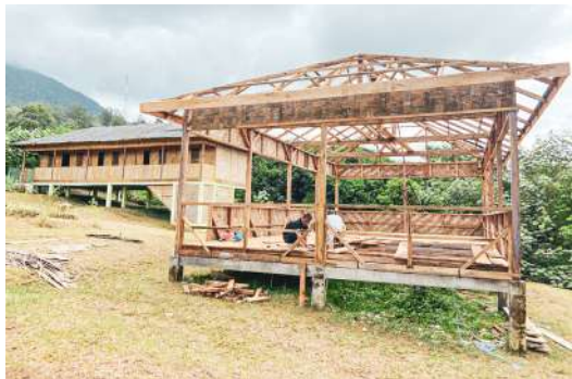
Construction of a multifunctional auditorium for children
