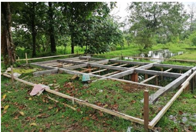
Foundations of the pondok above the pond
